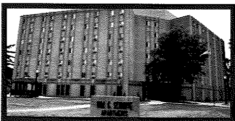
RAD I PROJECT #14-14 RENOVATIONS to William G. Schnute Towers Modernization of 115 units located in a 7 story High Rise. Located at 1030 W. Franklin Street, Evansville, Ind.
