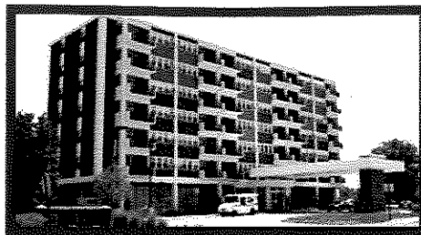
RAD I PROJECT #14-14 RENOVATIONS to George W. Buckner Towers Modernization of 108 units located in a 7 story High Rise. Located at 717Cherry Street, Evansville, Ind.
