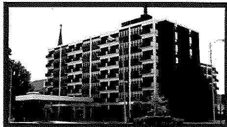
RAD I PROJECT #14-14 RENOVATIONS to John F. Kennedy Towers Modernization of 99 units located in a 7 story High Rise. Located at 315 SE Martin Luther King Jr. Blvd. Evansville, Ind.
